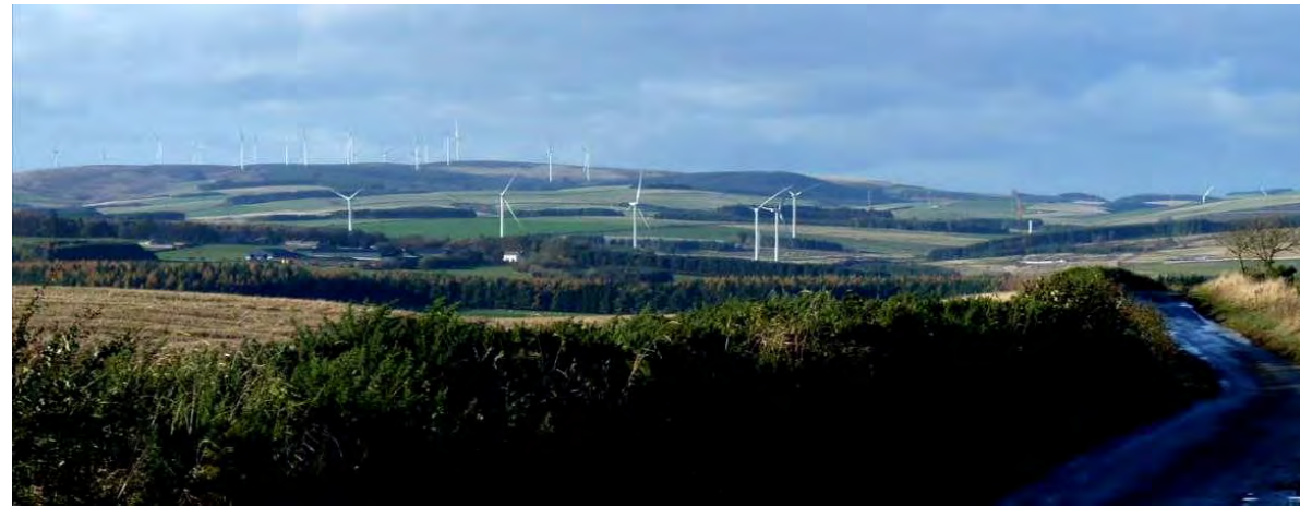
Eye Water Platform and Lammermuirs LCAs: Quixwood windfarm (under construction) in the foreground with Aikengall 2 and Crystal Rig in the background and Hoprigsheils just visible to the far right
